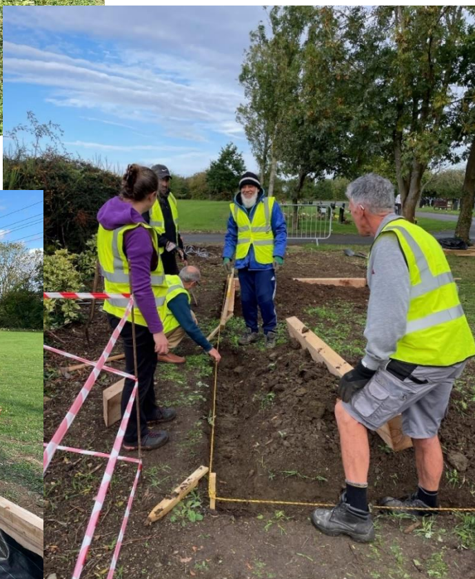
Below: Positioning the first bed along the marked out square.
